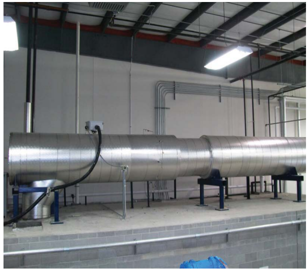
Figure 3: Aspirator in the inlet duct. Also shown are analyzer probes upstream.
